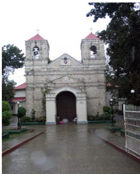
San Fernando Rey Parish Church of Liloan in Northeastern Cebu.
